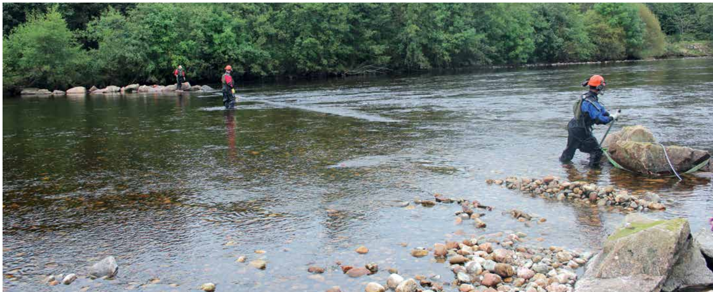
Figure 5. Croys being dismantled on the River Dee. © River Dee Trust.
