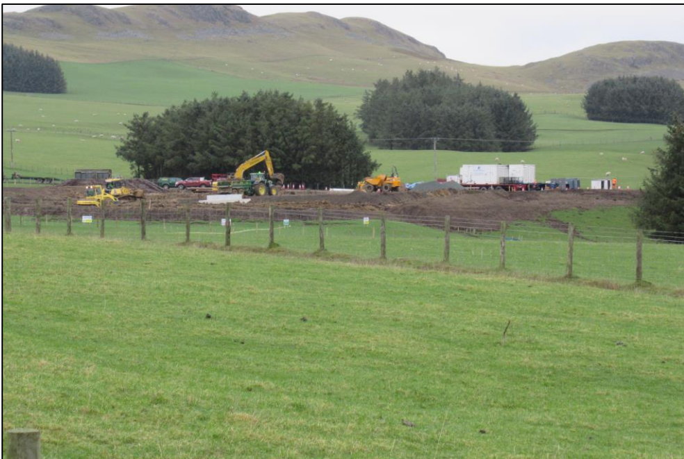
Figure 4. Site workings at turbine 5.
