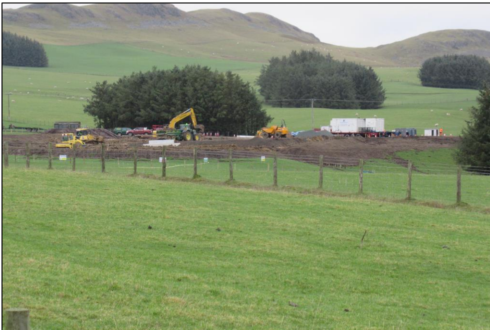
Figure 4. Site workings at turbine 5.
