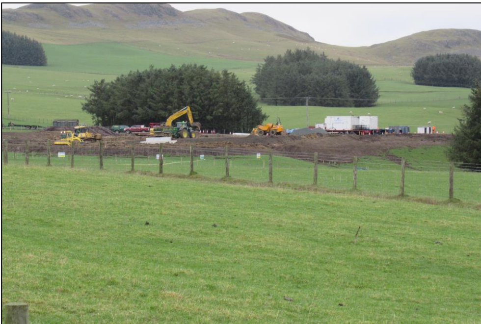
Figure 4. Site workings at turbine 5.
