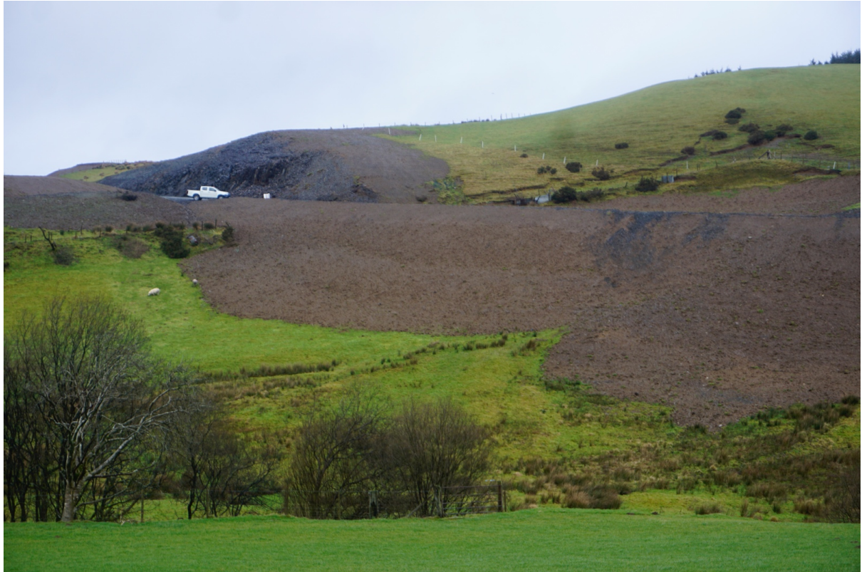
Access track with extensive cut and fill destroying wet-land vegetation and land-slippage
